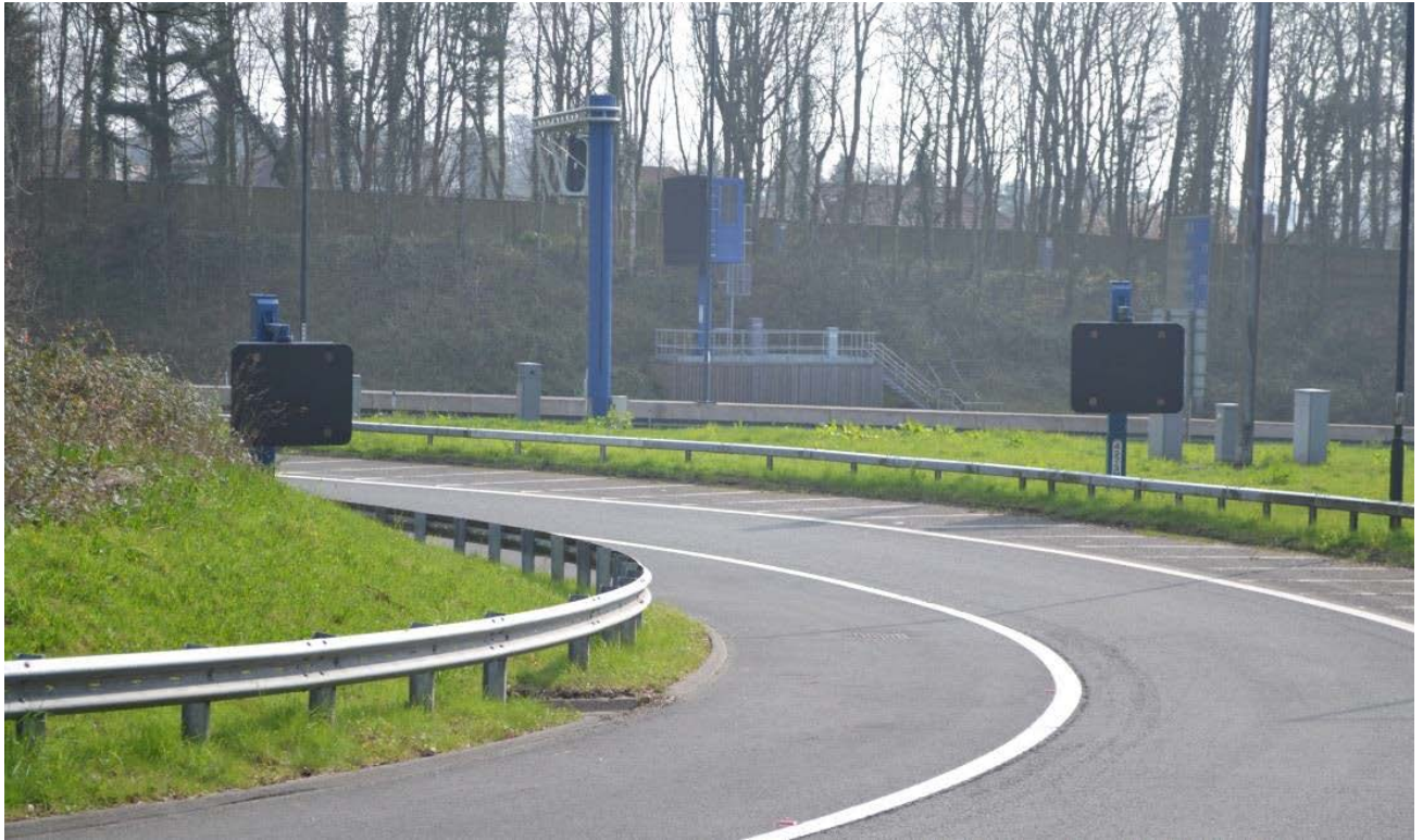
Figure 4 - Electronic signals on an entry slip road
