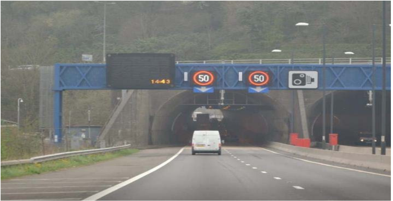
Figure 2 - Variable message sign at the side of the road and on an overhead gantry with speed limit signals
